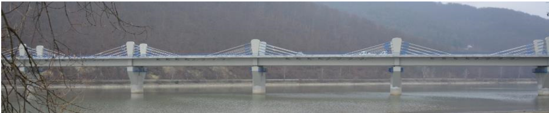
Nosicka dam railway extradosed 2-cell box girder bridge my last project in LKM consult; own work 100% on substructure and more than 85% on superstructure design. Actually finished construction (2021)
