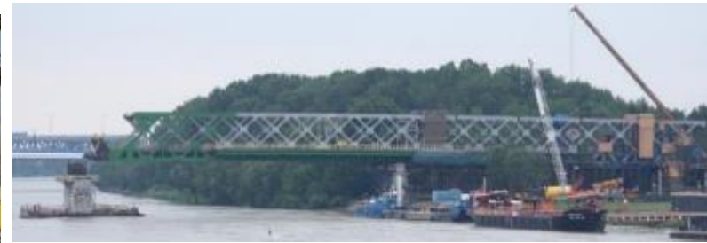
Nosicka dam railway extradosed 2-cell box girder bridge my last project in LKM consult; own work 100% on substructure and more than 85% on superstructure design. Actually finished construction (2021)
